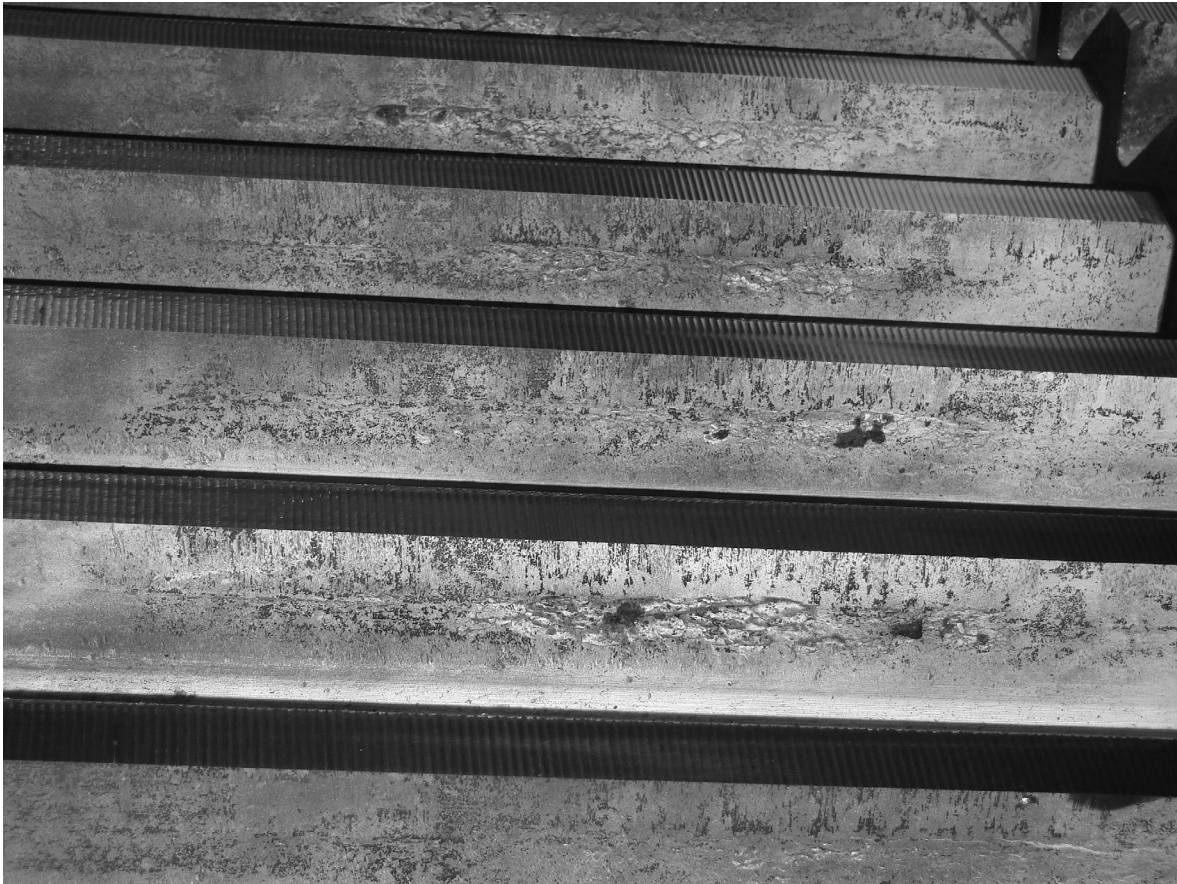
Picture 1 Typical misalignment damage on a girth gear
