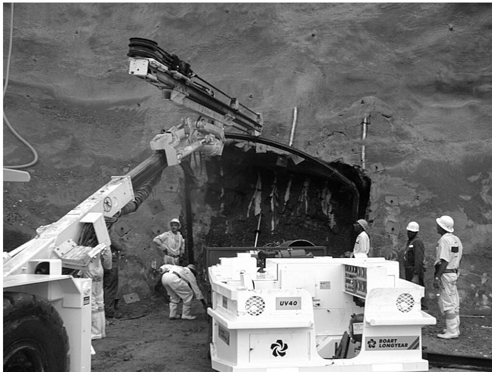
Figure 1. Wet shotcreteing used to support a new decline.
