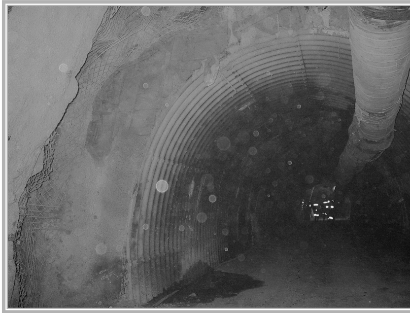
Figure 16. Void Filled with Aerated Cements.
