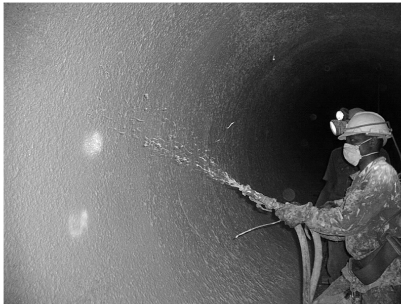
Figure 14. Supporting of a raise bore hole with a TSL
