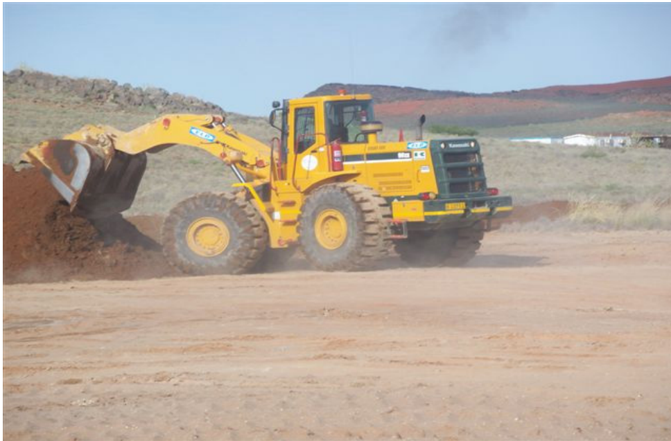
Figure 6.3: Rehabilitation of earth dams in progress
