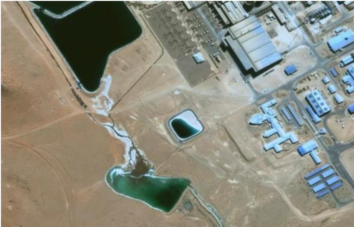
Figure 4.1: Filled evaporation pond and overflow to earth dams
